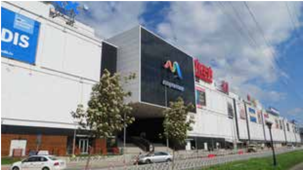
Sochi More-Mall Centrifugal Chiller Russia
