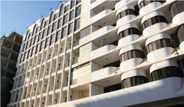
Trading Building Air Cooled Screw Chiller Oman
